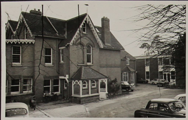
The front - showing the new Casson Wing.
