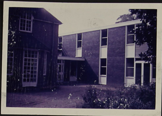
The front entrance
