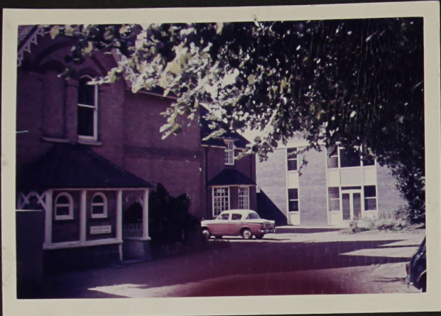
The front - showing the new Casson Wing.
